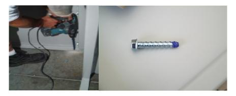
Insert the rear concrete anchor Wedge Bolts illustration # 5 and tighten evenly "do not over tighten" With the shelter fully open locate & drill the holes for front anchors using 5/8" concrete bit and hammer drill. Insert the front concrete anchors and tighten evenly "do not over tighten". Clean area after drilling to remove concrete dust and debris.
