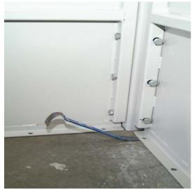
Remove all shims and test door opening & closing, adjust door so it clears floor by 1/8" and does not drag against the floor.
